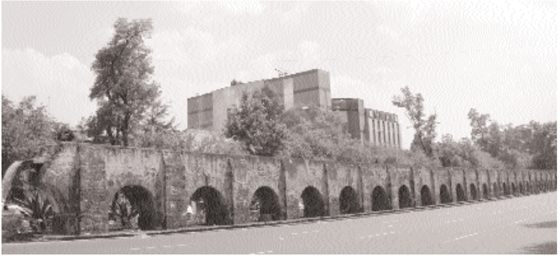
9.4 Remains of the aqueduct that carried freshwater from Chapultepec to Tenochtitlan (Fernando González y González)
